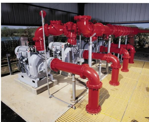
The pump isn't re-priming as rapidly as it once did. Most commonly, slower re-prime can be attributed to excessive face clearance. If this is not the cause of your slowdown, check the following:
